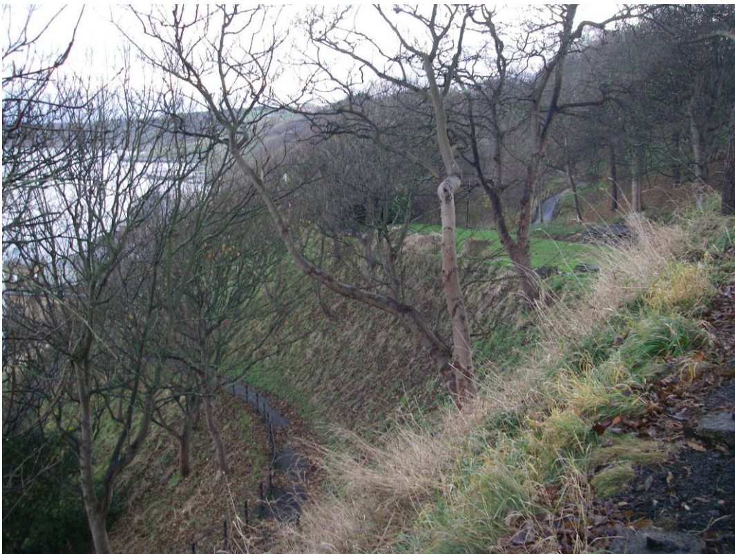
Plate 28 Site view looking south across Spa Cliff showing steep slope angles and bench-cut paths.
