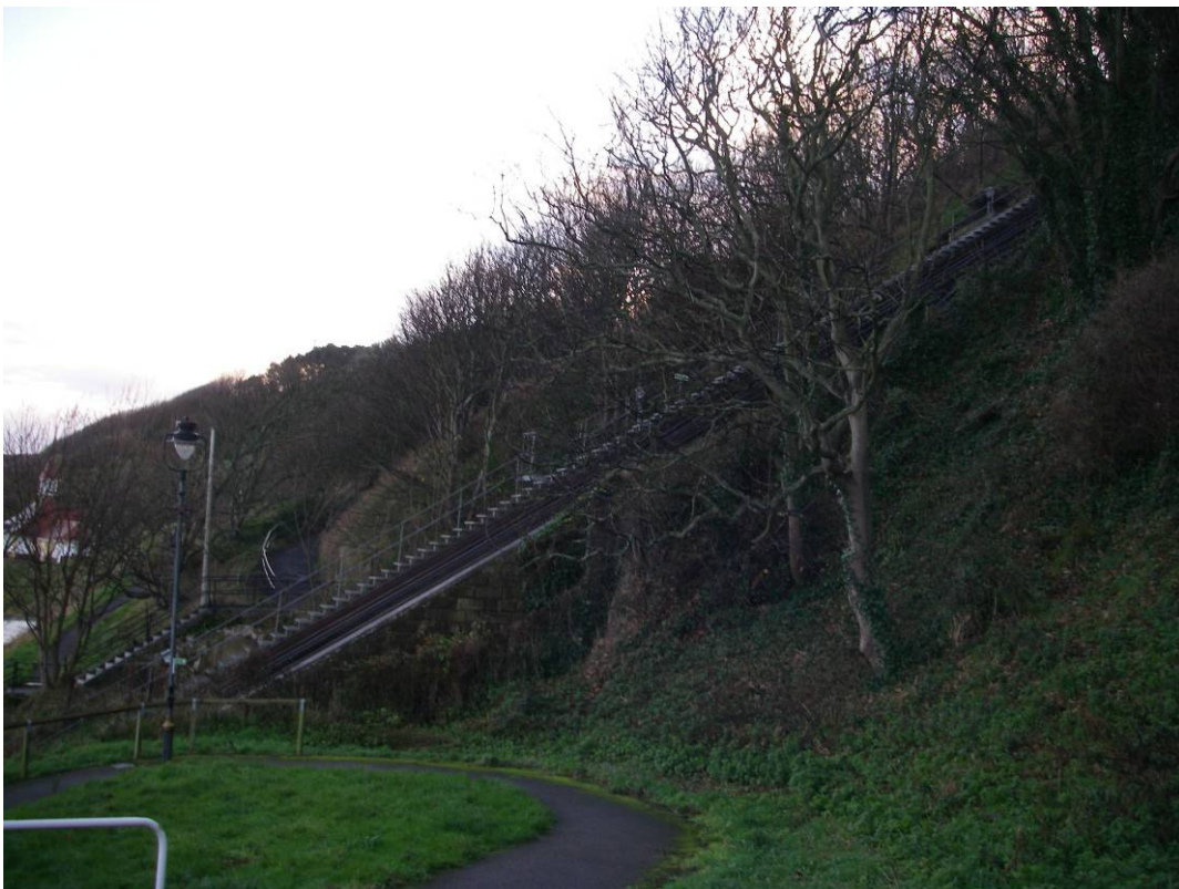
Plate 26 Site view looking south at the cliff railway and slopes of Prince of Wales Cliff.
