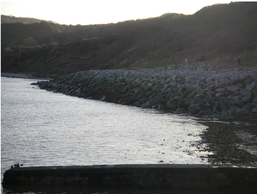
Plate 4 Site view looking south-south east across rock armour revetment towards Dother Pits.
