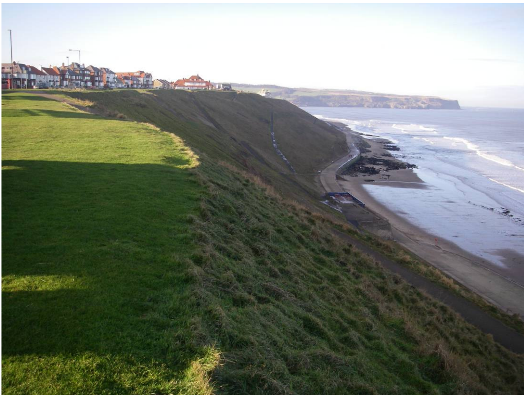
Plate 6 Site view looking west along West Cliff towards Sandsend.
